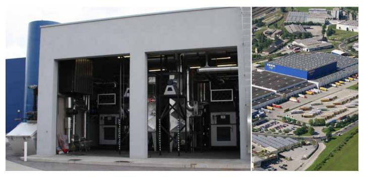
The Ikea name speaks for itself. It uses Froling technology to heat many of its premises. At its central warehouse in Wels 2x 1,000 kW boilers provide heat from pellets.
