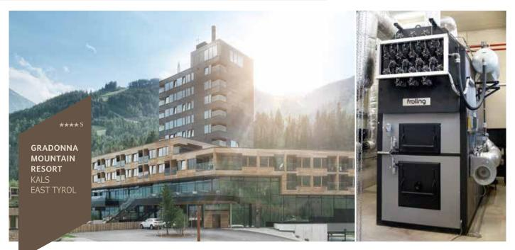
A Froling cascade system provides cosy warmth from wood at the four star superior Gradonna Mountain Resort hotel in Kals am Großglockner, Austria. The specification was to find a solution that would be able to handle a wide range of fuel qualities (dry/wet, small/large) as efficiently and as reliably as possible. Fabric filters were included to ensure optimum cleaning of the flue gas and a condenser unit was integrated to increase energy efficiency.
