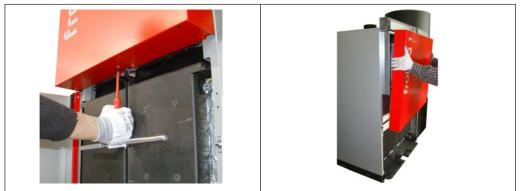
Remove the screw and contact washer on the bottom of the controller cover
