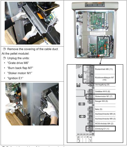
Pull out the cables of the unplugged units
